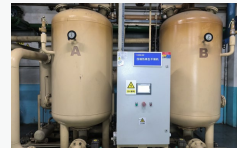
Compressed Air System Retrofitting at Shenyang Factory
